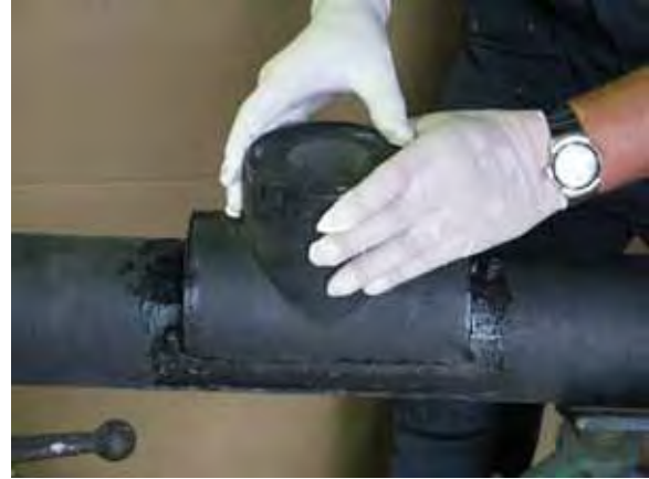
Figure 31 Setting the saddle
