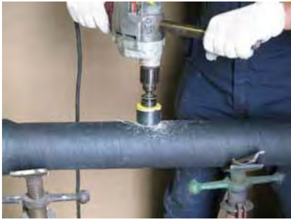
Figure 24 Drilling the branch hole
