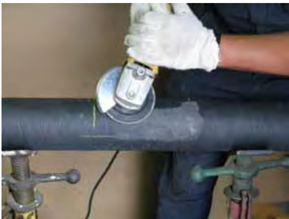
Figure 25 Sanding the pipe
