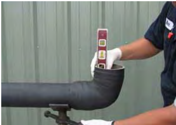
Figure 17 Checking plumb
