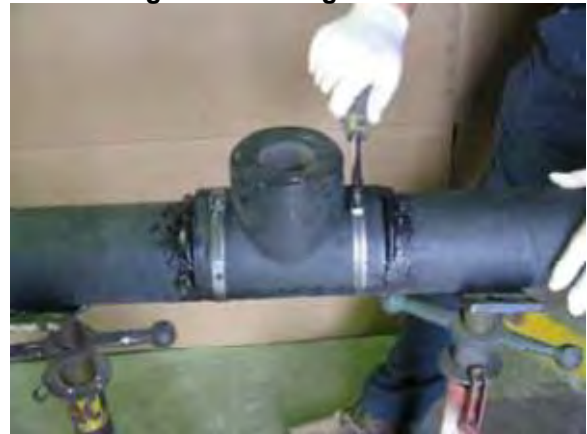
Figure 32 Securing the saddle and squeezing the adhesive
