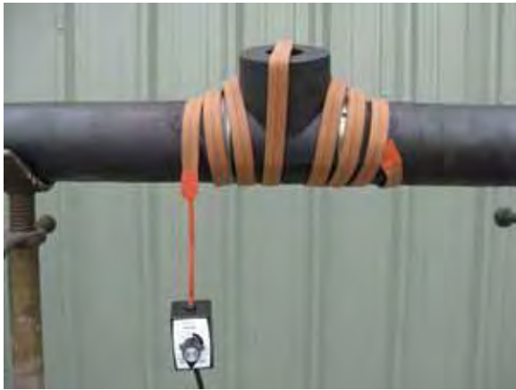
Figure 33 Heat tape curing
