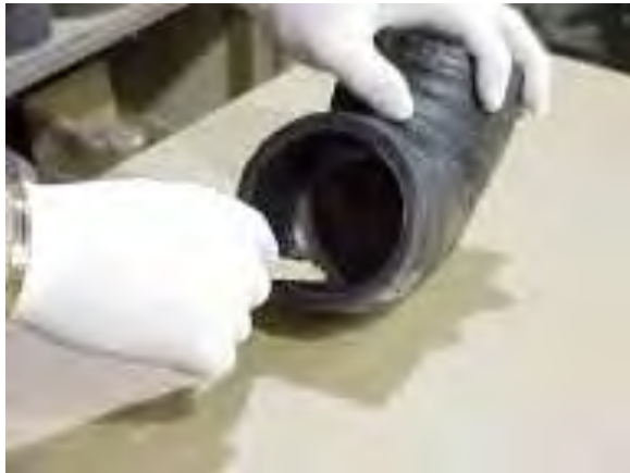
Figure 12 Even coat of adhesive in the socket
