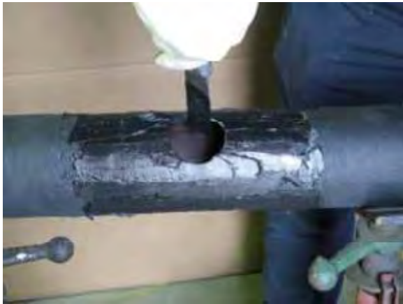
Figure 29 Sealing (scrubbing-in) the branch hole
