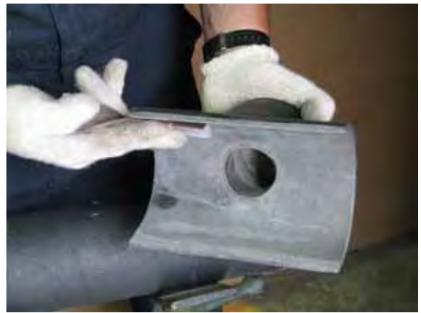
Figure 26 Sanding the saddle
