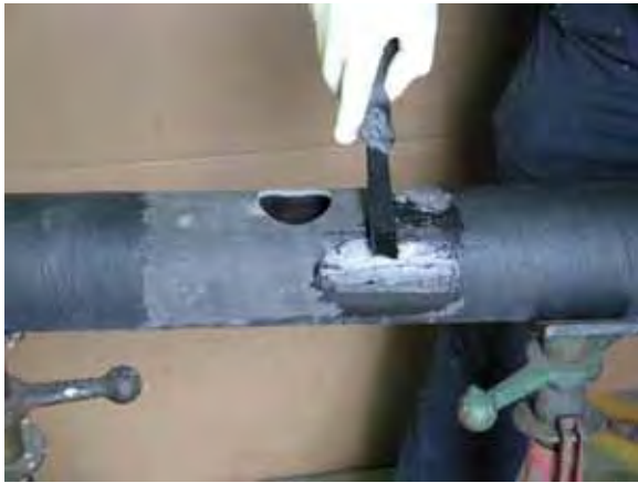
Figure 28 Scrubbing in the pipe surface
