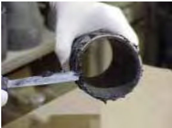
Figure 8 Scrub the end of the pipe
