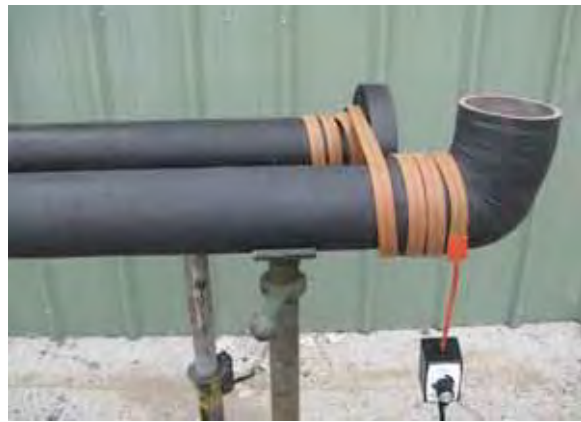
Figure 21 Do not overlap heat tape.
