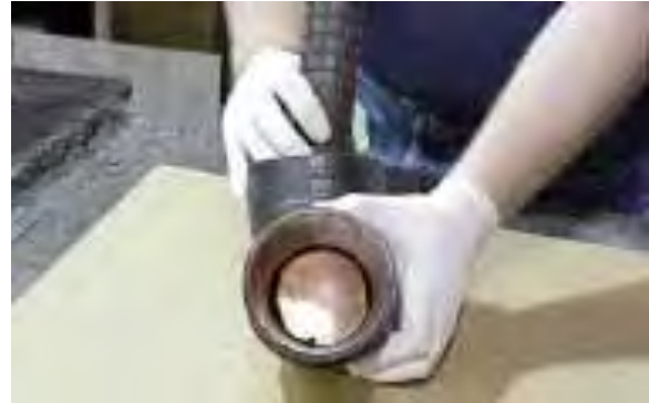
Figure 19 Visually inspect for the correct amount of adhesive, a small even bead
