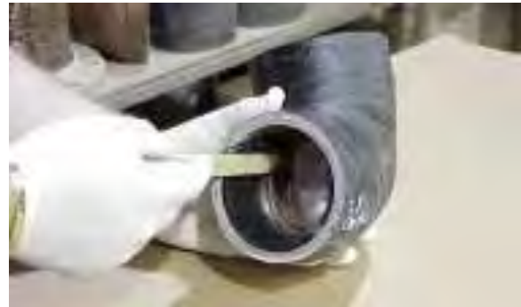
Figure 10 Scrub the socket of the fitting
