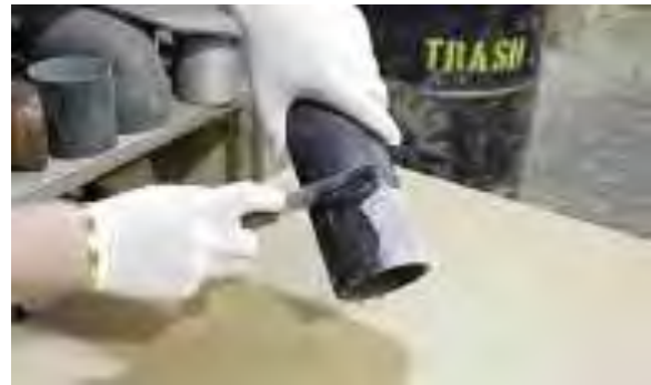
Figure 9 Scrub the sanded surface of the pipe
