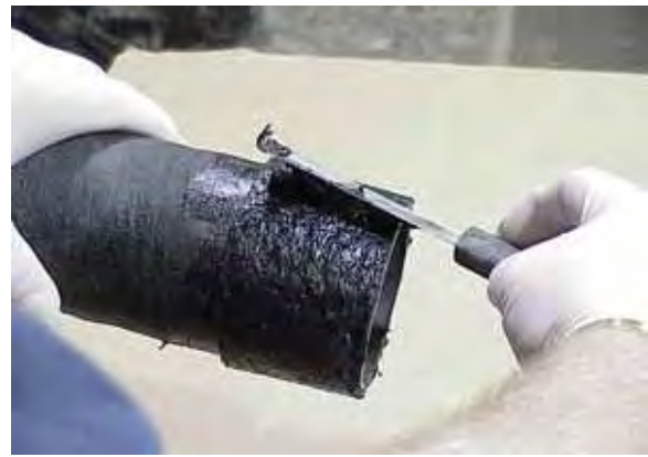
Figure 13 Applying adhesive
