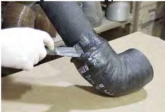
Figure 18 Pulling a fillet
